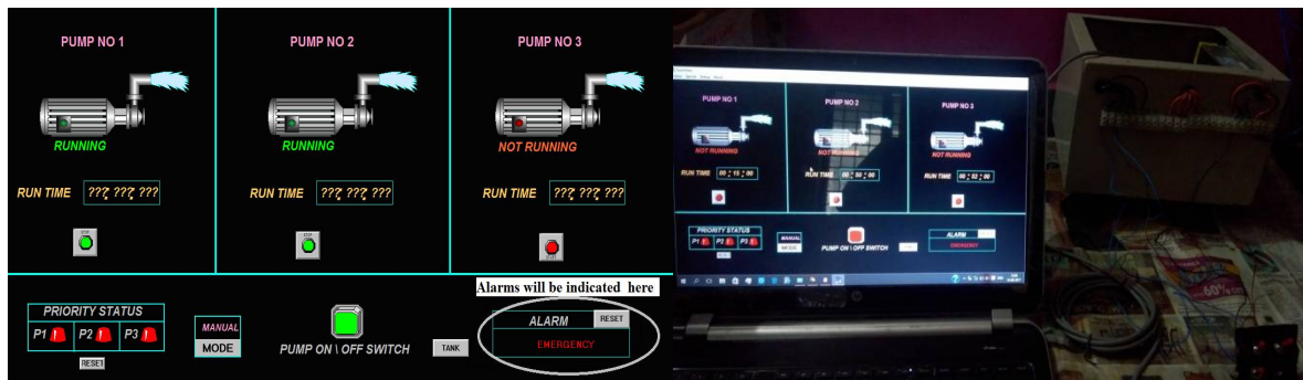
Fig 7 Fault indications by SCADA
