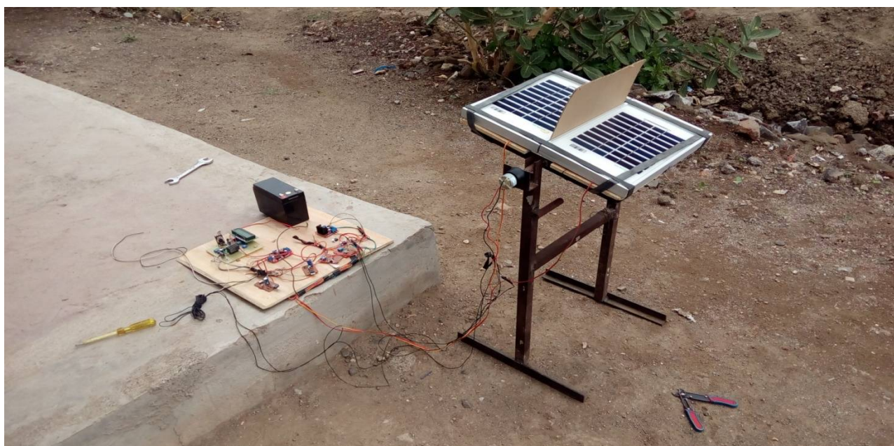
Fig.1 solar tracking system.
