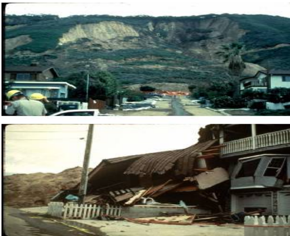
Figure 2.1. Landslide and loss due to it.
