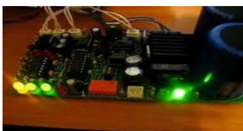
Figure No 3: Voltage monitoring unit
