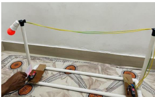
Fig.6 Turning on the overhead lines using RF Card
