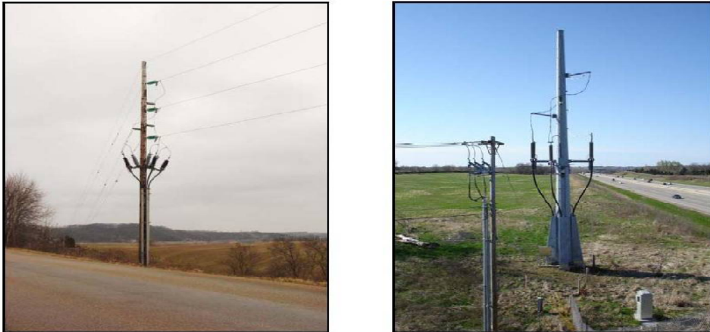
Figure.3.1 overhead to underground transmission structure.
