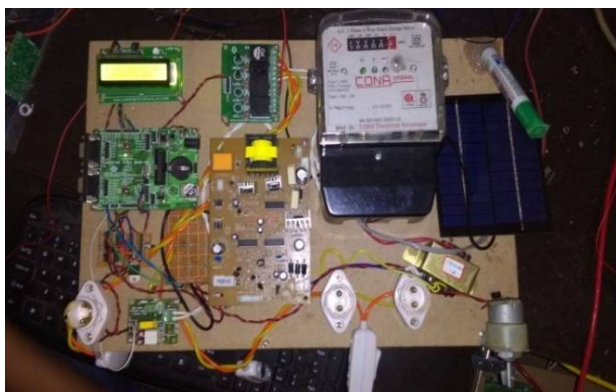
Fig. 3. Smart Energy System Installation
